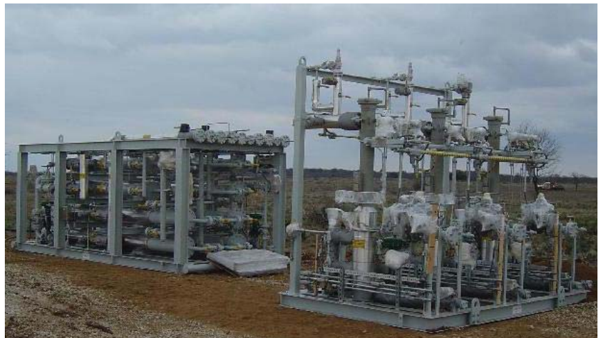
Installation of a wellhead N 2 removal system
