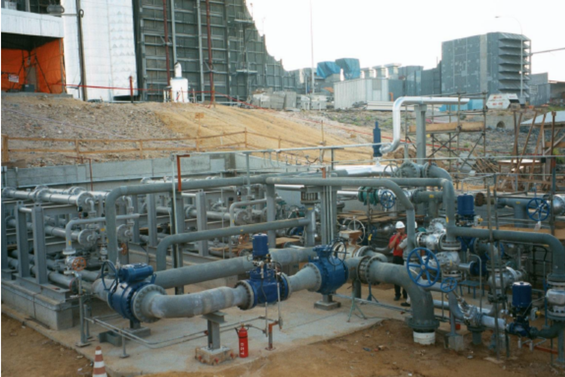
Figure 8. Photograph of a membrane unit for conditioning turbine fuel by removing hydrocarbons.
