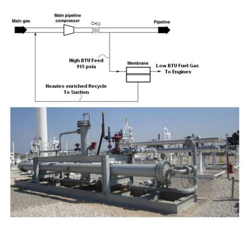
**Figure 2.** Block diagram and photograph of a membrane FGCU used for a gas gathering compressor engine in the Eagle Ford Shale, TX. The membrane modules are contained in the horizontal pressure
